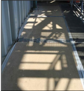
Plywood Flooring in the Containment Area
