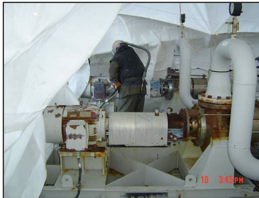
Water Blasting Showing Containment Structure and PPE
