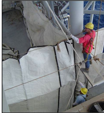
Blast Abrasive External Containment Being Installed
