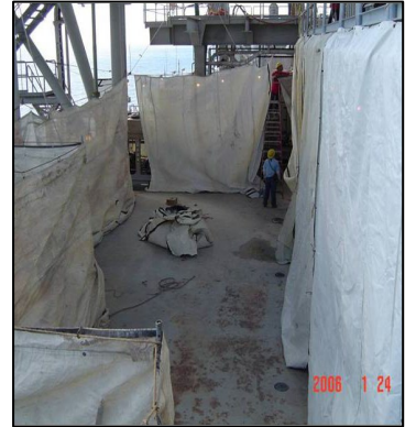
Blast Abrasive External Containment Being Installed II
