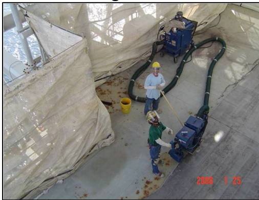
Blast Abrasive External Containment
