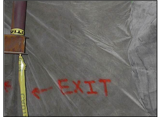
Overlapping Walls with Designated Exit from the Blasting Area II
