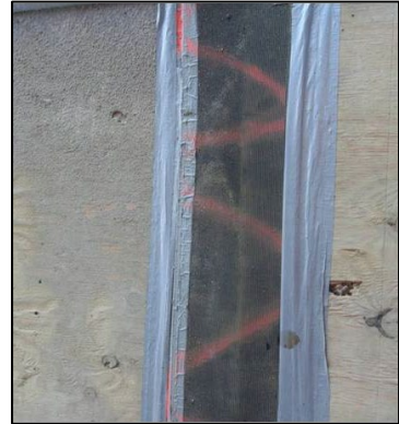
Close-up of Sealed Joints between Plywood Flooring in Containment Area
