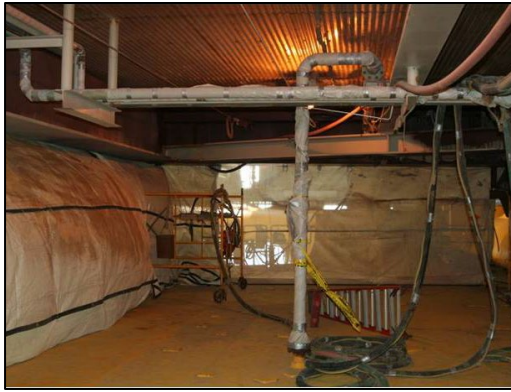
Blast Abrasive External Containment III
