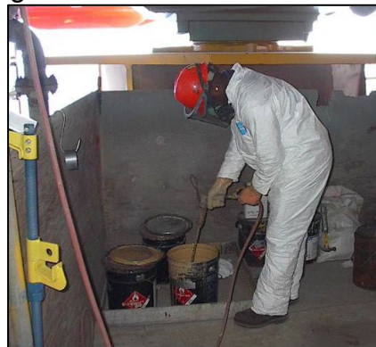
Paint Containment Structure II
