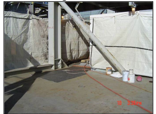
Blast Abrasive External Containment II
