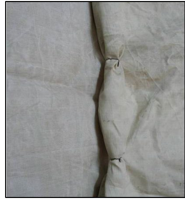
Overlapping Containment Wall Secured Together in the Blasting Area
