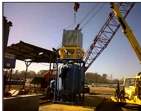
New, Unused Blast Abrasive Being Transferred from Hopper to Blast Pot
