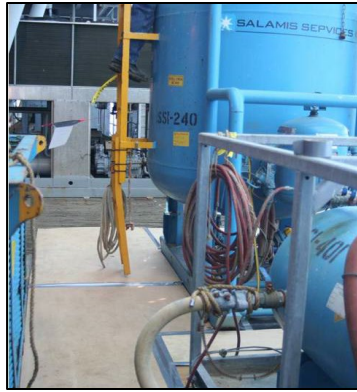
Containment Below the Blast Abrasive Pressure Vessel
