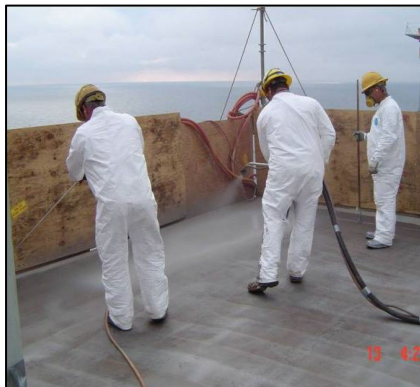
Painting in Contained Area
