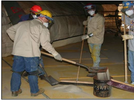
Collection of Spent Abrasive in Containment Area
