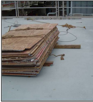
Plywood Flooring for Containment Area
