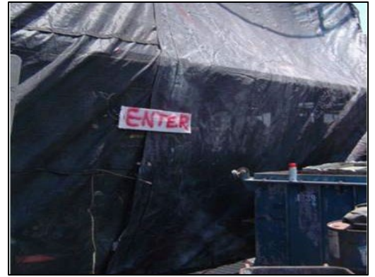
Overlapping Walls with Designated Entrance to the Blasting Area
