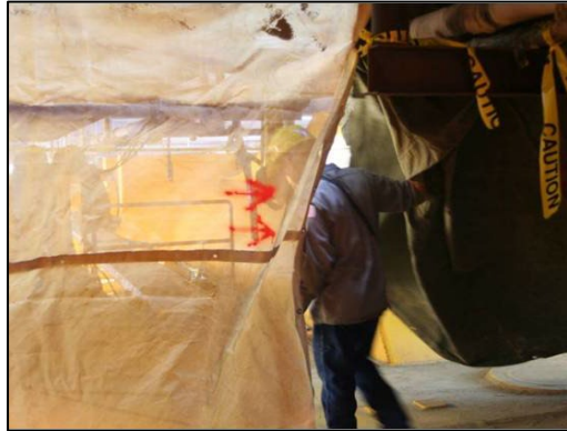
Overlapping Walls with Designated Exit from the Blasting Area
